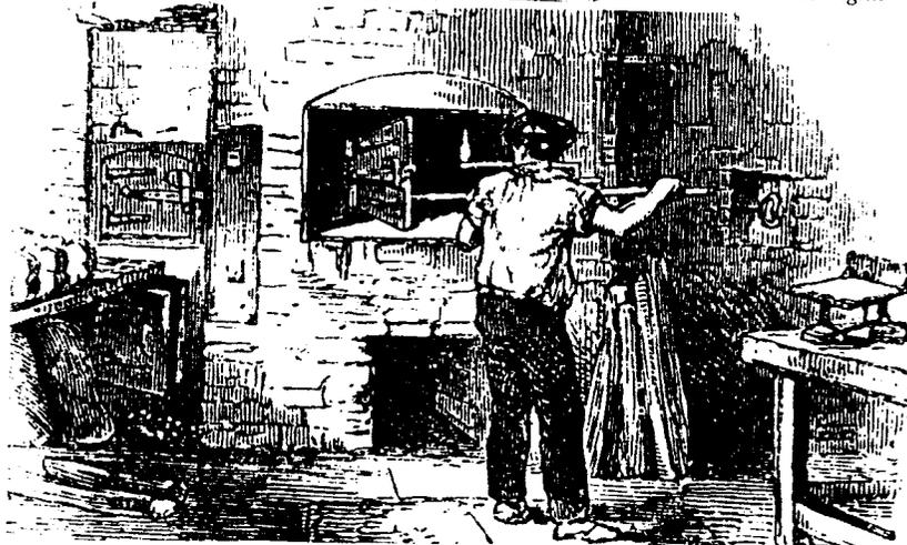
BELOW: *The side flue oven of about 1830. The fire door is on the left of the oven, the draught is adjusted by the handle on the right.*
