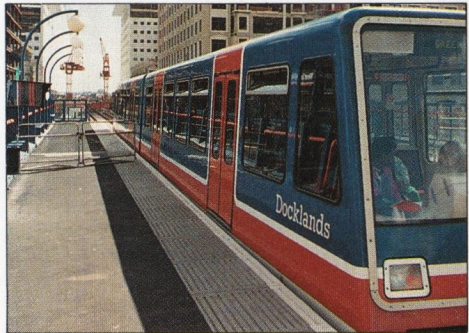
Longer platforms: (West India Quay Station)
