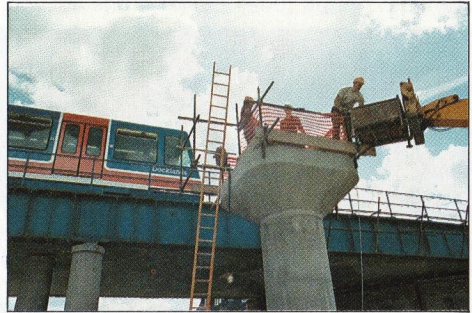
Construction at West India Docks
