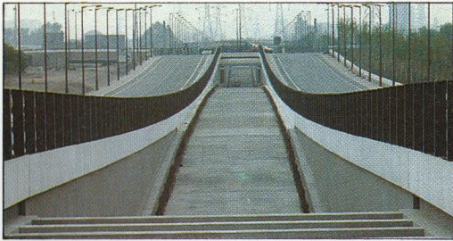
Construction at Beckton
